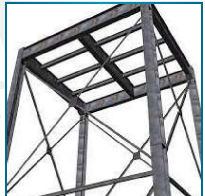
Water Tank Structure
